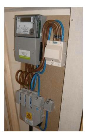
6. Once the metering has been installed, setup and tested by IMServ a new connection form will be provided to the customer. The metering will be installed by IMServ with an isolator ready for the customer's electrician to connect to. IMServ technicians will not connect metering directly to customers installations this final connection must be done by an approved electrician arranged by the customer.
