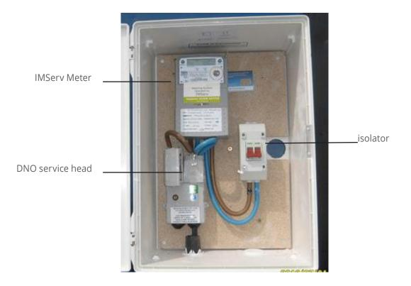
5. Three phase supply after meter installation:
