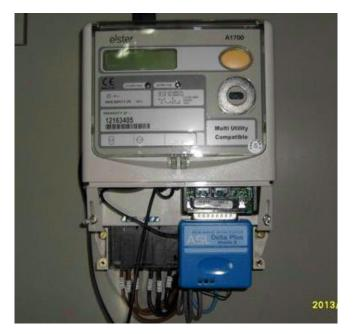
**5.** If the supply is fed from a DNO cut out (generally up to 600 amp), the fuse holders are present and all wiring between cut out, CT chamber and customers main switch has been completed by the DNO and the customer's electrician. IMServ will energise the supply up to the main switch.
