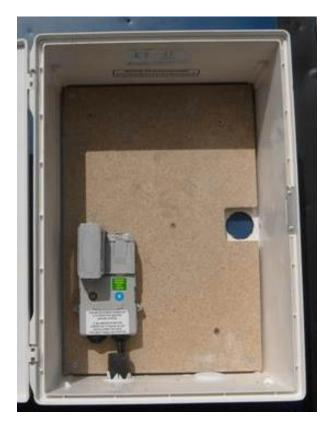
**3.** Three phase supply ready for new connection; cut out is installed by and is the property of the DNO (please note supply must be live up to the cut out/service head or the meter cannot be installed):
